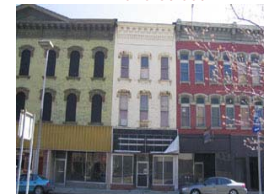
112 Lake Street 1,400 Square Feet
