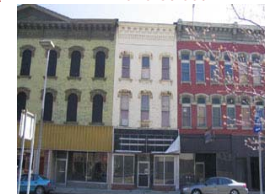
112 Lake Street 1,400 Square Feet
